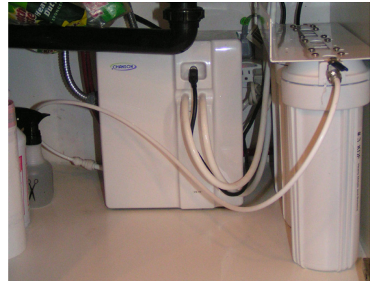
Pictured with the Chanson VS-70 Undercounter Ionizer. H3 Pre-Filter is on the right.
